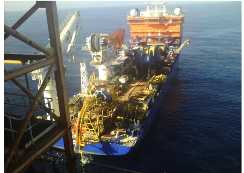
CSV Southern Ocean at GWF field Australia laying umbilical
