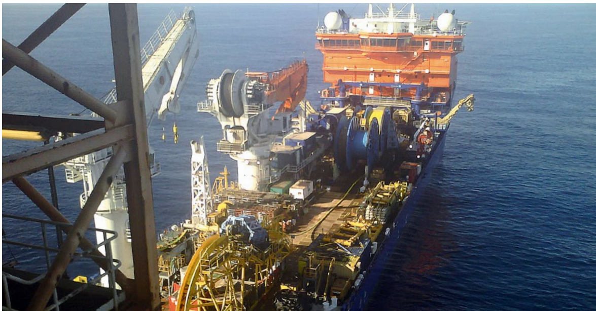
CSV Southern Ocean laying umbilical at GWF field, Australia
