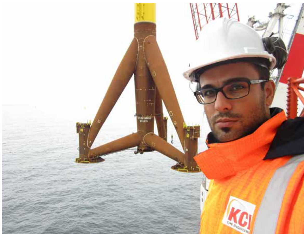
KCI monitoring of tripod installation for offshore windfarm Global Tech I.
