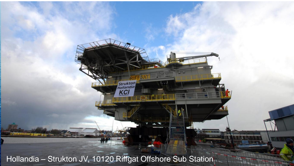
Wintershall, Relocation of MPP P6-S to Q1-D
