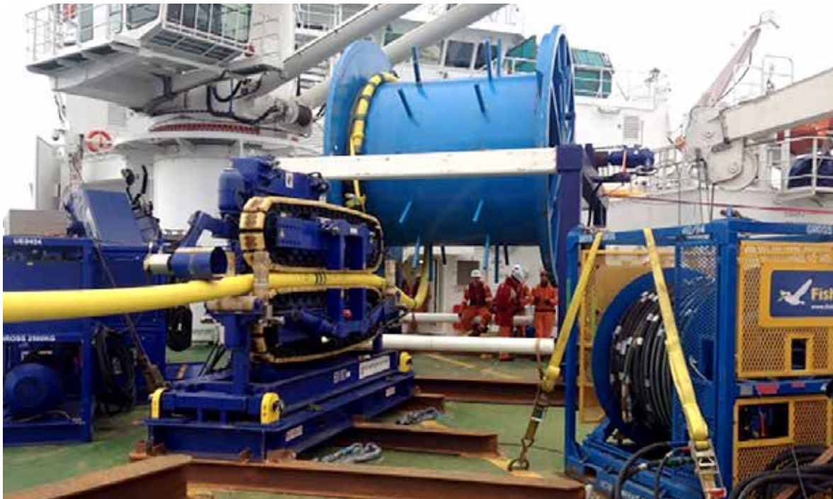
Installation of gas export flexible in The Netherlands
