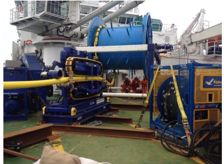
Installation of gas export flexible in The Netherlands
