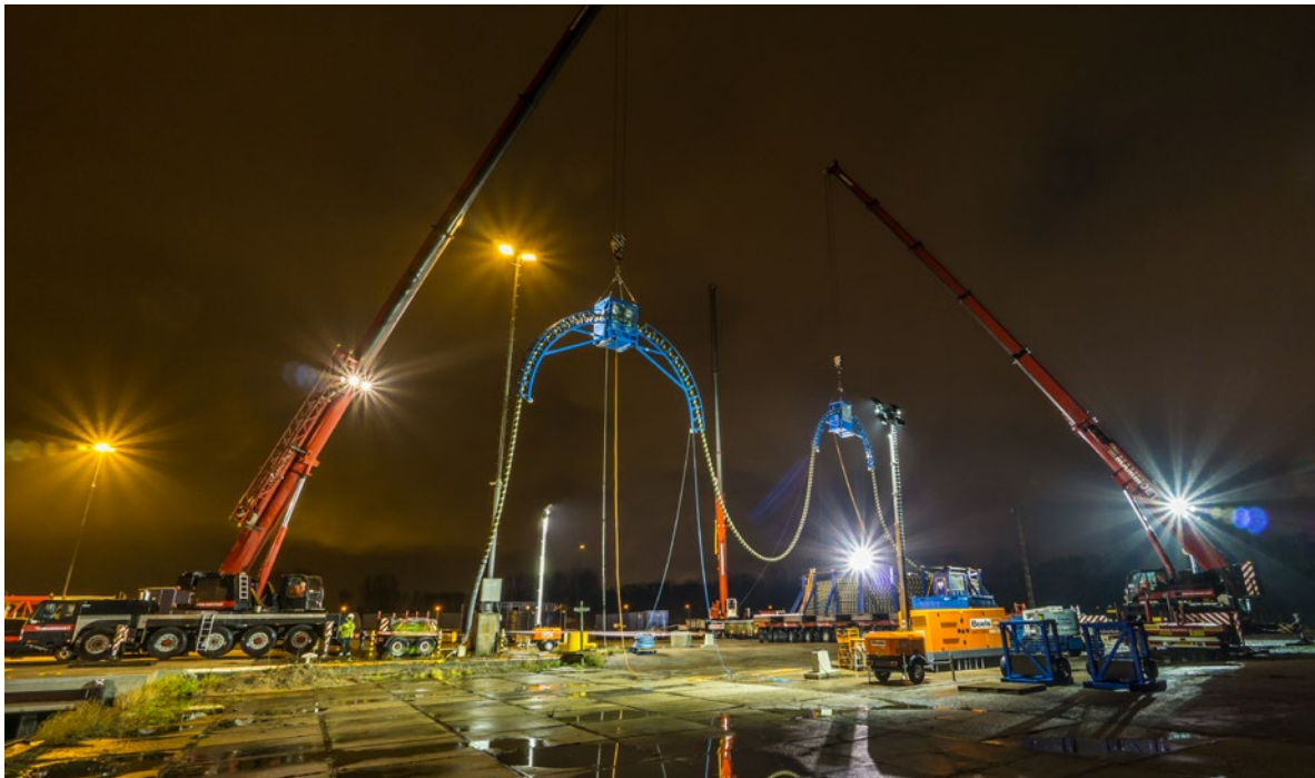
Oceanteam Solutions successfully performed cable loadout at Velsen Noord base
