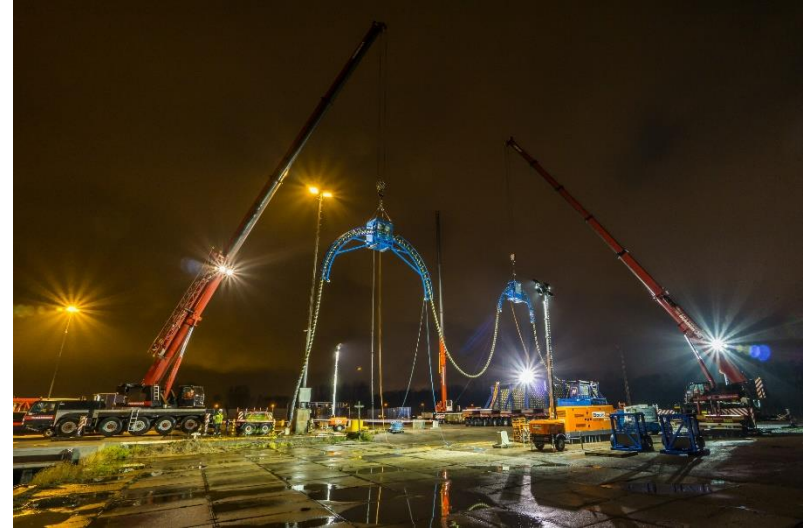
Oceanteam Solutions successfully performed cable loadout at Velsen Noord base
