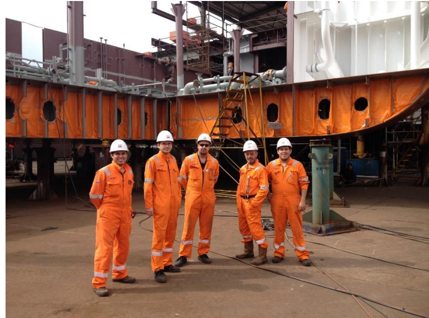
Part of the team working on construction of Tampamachoco I
