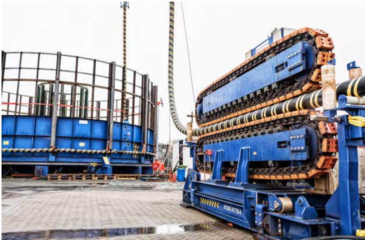
Transpooling of cable at Oceanteam's storage facility in Velsen Noord, the Netherlands
