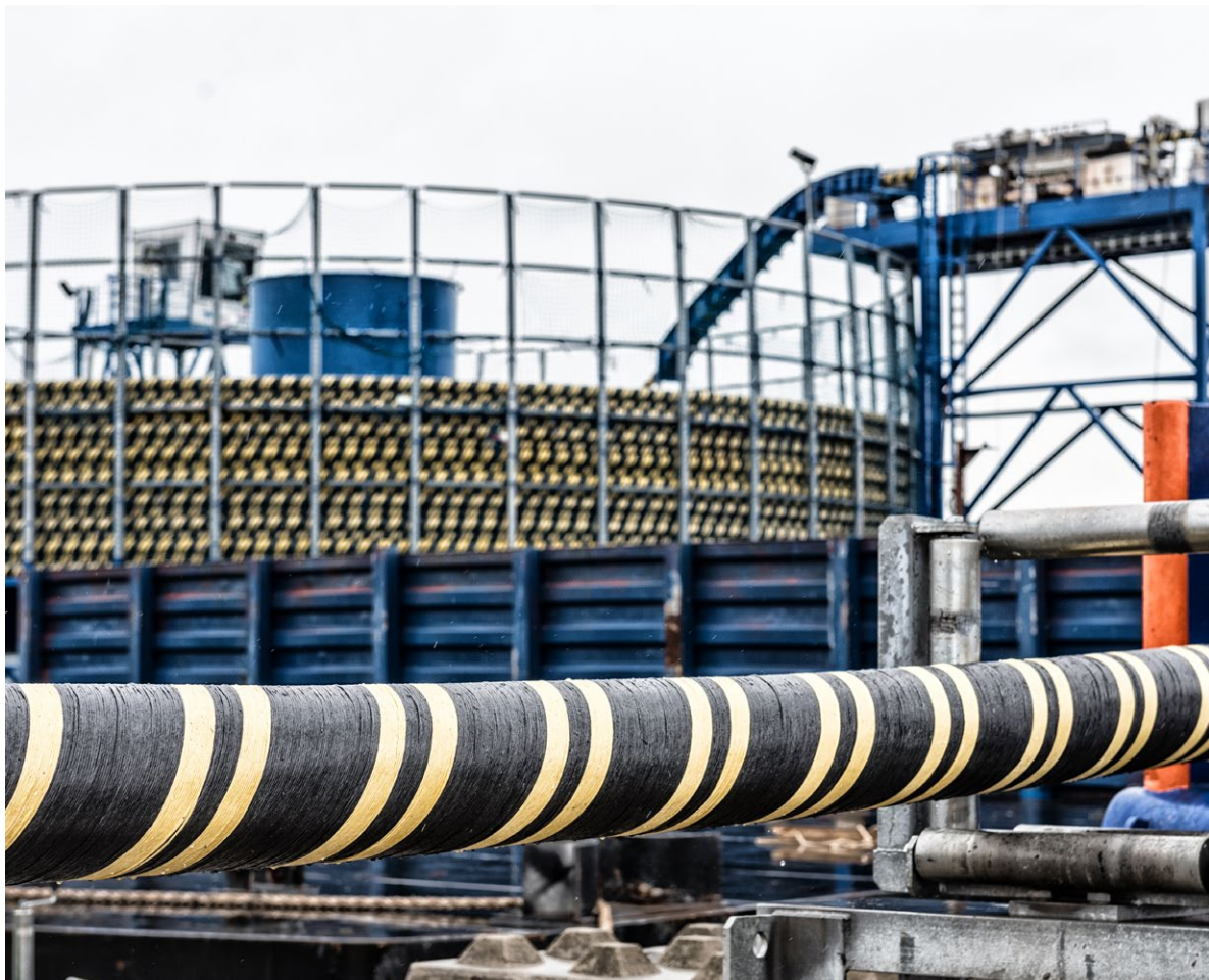
Transpooling of cable to Oceanteam's 1100t turntable.
