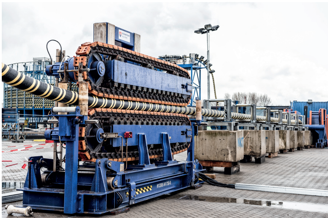
Spooling operations at cable storage facility Velsen, the Netherlands
