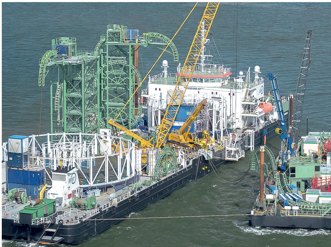
Oceanteam's 4000Te and 2000Te carousels during cable installation works
